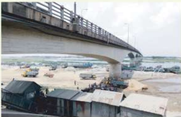
Land Alignment for 2nd Bridge Construction on Meghna River
