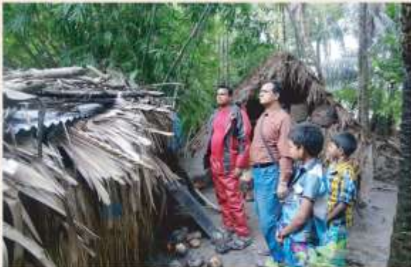
Staff Surveying Damage after Cyclone Mahasen
