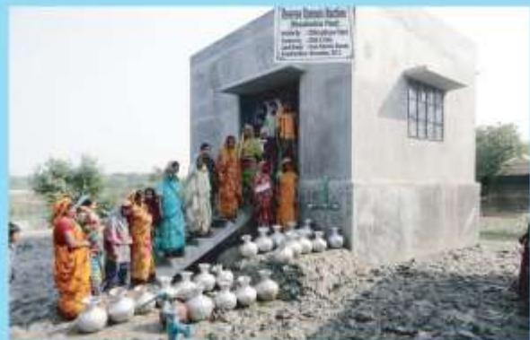
Reverse Osmosis Plant in Saline Prone Area
