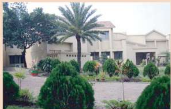
CCDB-HOPE Foundation Accommodation Building
