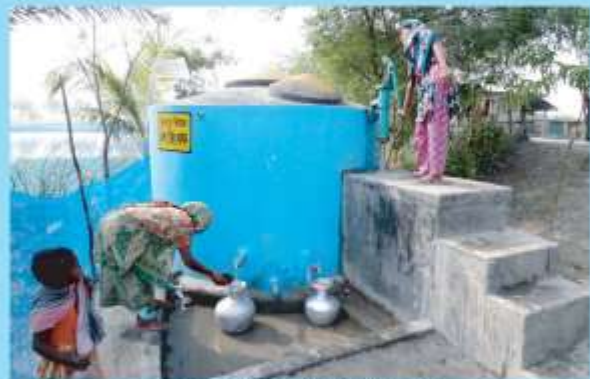
Pond Sand Filter for Safe Drinking Water
