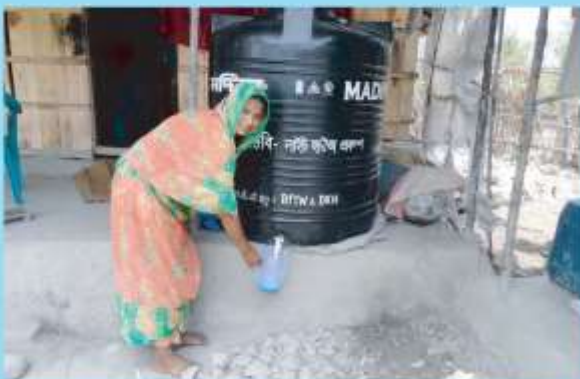
Household Level Rain Water Harvesting
