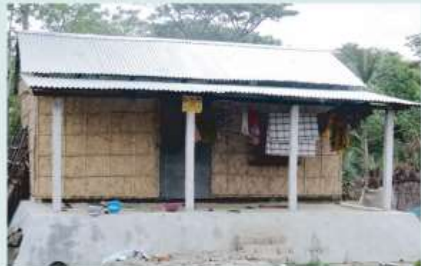
Building Fortified Cyclone Resistant Houses
