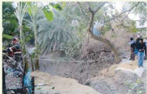
Measuring Small Scale Water Resource Canal Reexcavation for Irrigation
