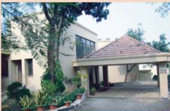
CCDB-HOPE Foundation Reception Block
