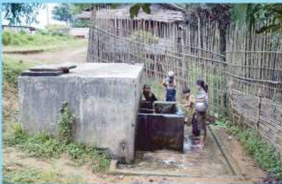
Gravitational Force Water Collection in Bandarban
