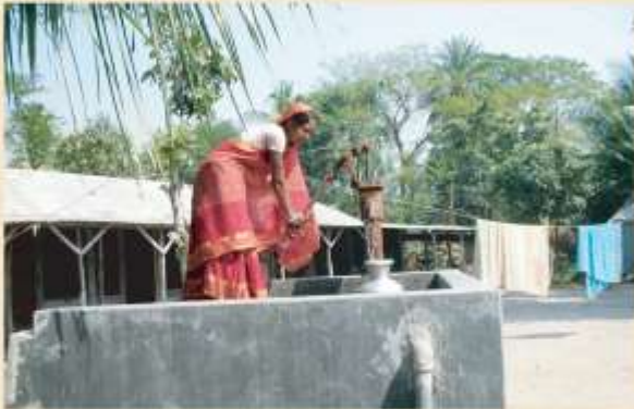
Tubewell Plinth raised about Flood Level
