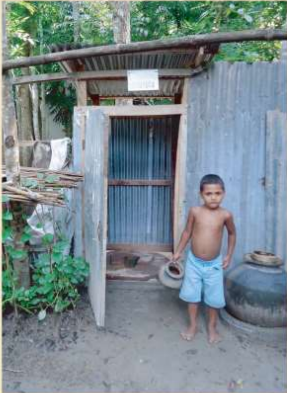
Using Ring Slab Latrine
